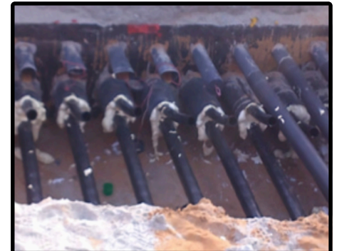
Cable duct Bentonite Filling
